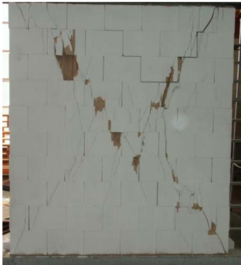
figure A2-1: crack pattern of test No. 2
