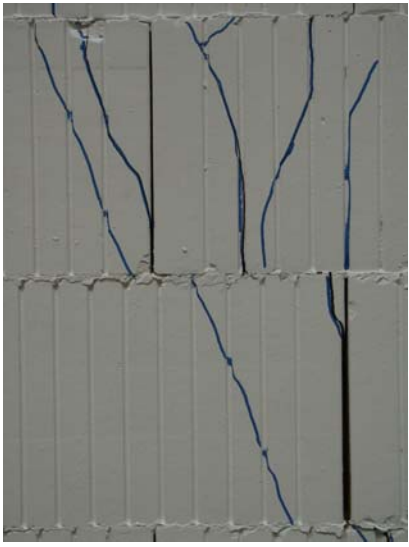
figure A12-2: detail of the crack pattern of test No. 12
