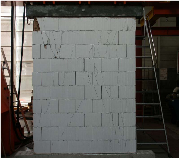
figure A3-2: crack pattern of test No. 3
