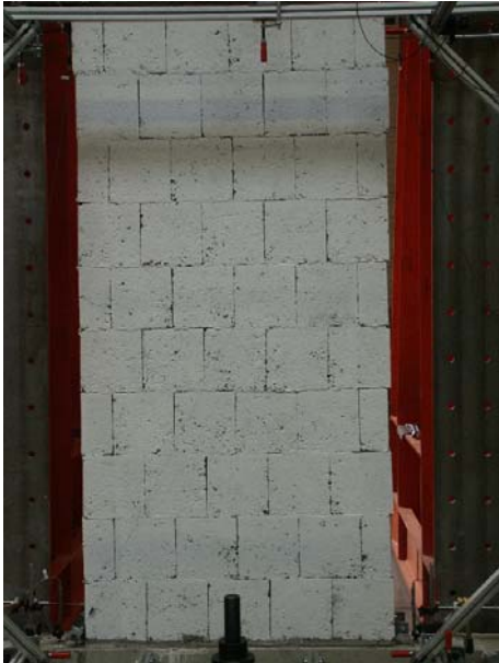
figure A21-1: crack pattern of test No. 21
