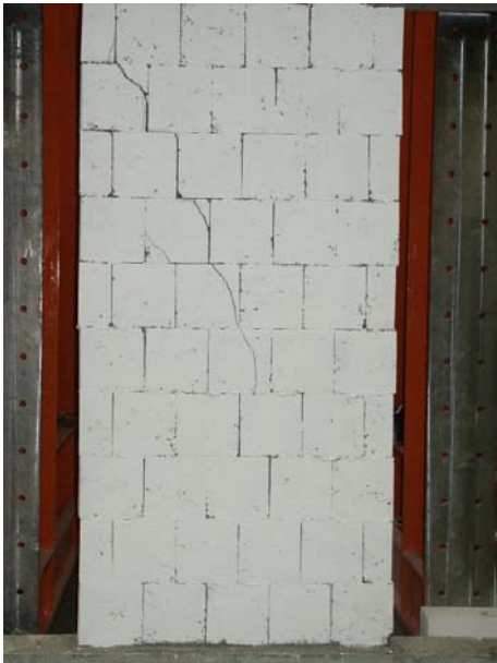
figure A19-1: crack pattern of test No. 19
