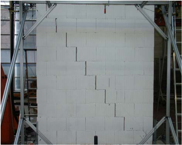
figure A9-2: crack pattern of test No. 9
