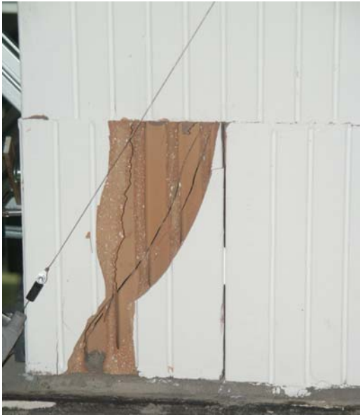
figure A7-2: local failure of wall No. 7
