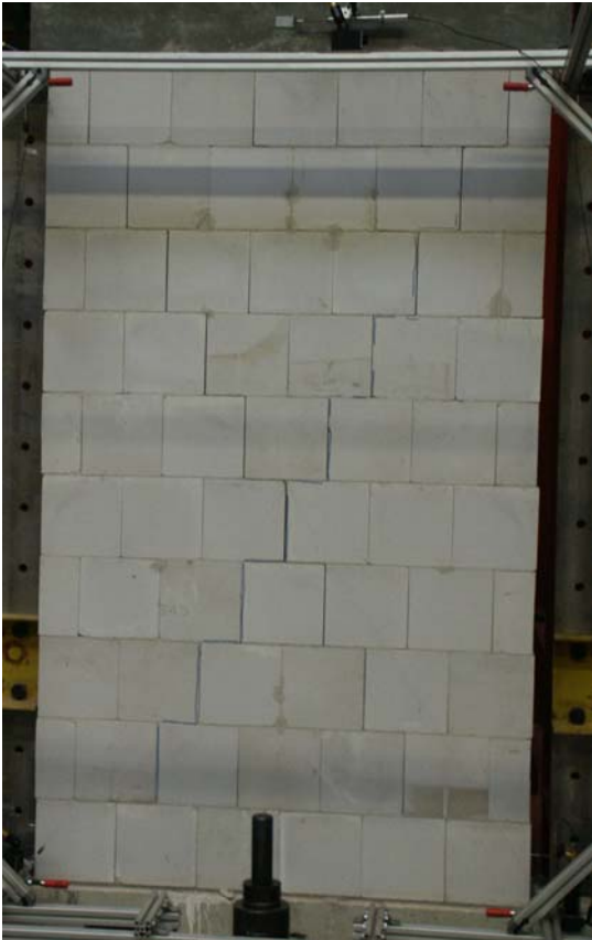
figure A4-1: first cracks at about 35 kN of wall No. 4
