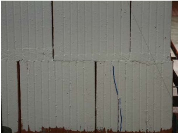
figure A8-2: crack pattern of wall No. 8
