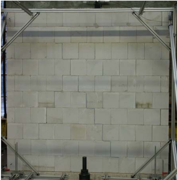
figure A3-1: first cracks at about -75 kN of wall No. 3
