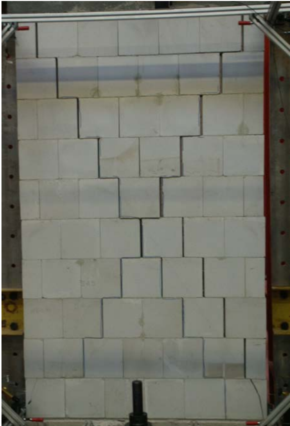
figure A4-2: crack pattern of wall No. 4 (predamaged)
