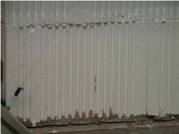
figure A6-1: opening of the bed joint of wall No. 6
