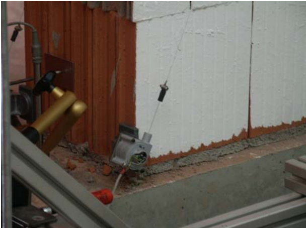
figure A8-1: gapping of the bed joint of wall No. 8
